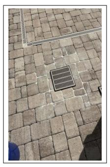
RMS re-leveled pavers on the pool deck, reset the drain, and cleaned out debris in the catch basin to allow better flow of water during heavy rains. RMS also replaced the broken entry handle to the Amenity Door.
