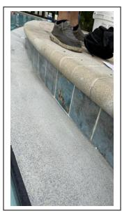
CBuss completed the necessary repairs to the broken and missing tiles on the pool deck.
