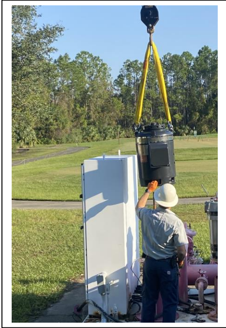
M&M Pumps installed (2) new irrigation pumps at the pump station.
