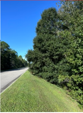
OVERGROWN WOOD-LINE HEADING TO 100 ENTRANCE
