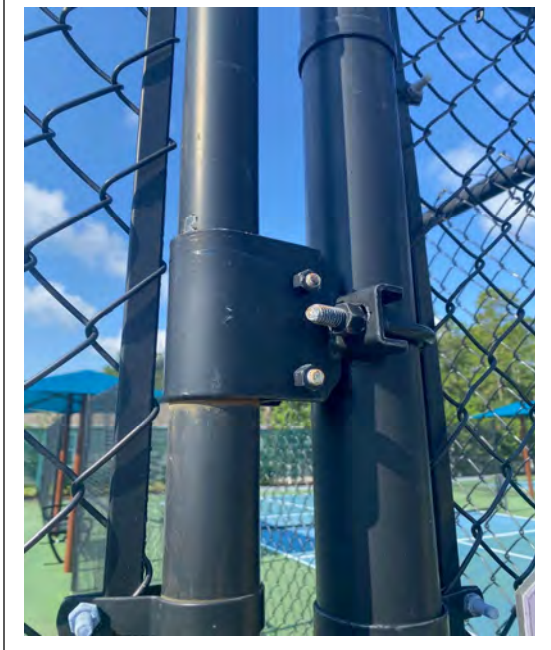
RMS staff installed Automatic Door Closures on all (4) Pickleball Entry Gates
