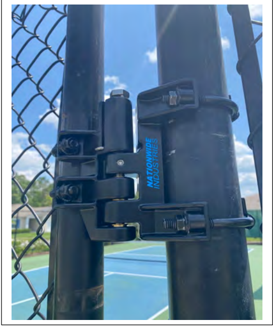
RMS staff installed Automatic Door Closures on all (4) Pickleball Entry Gates
