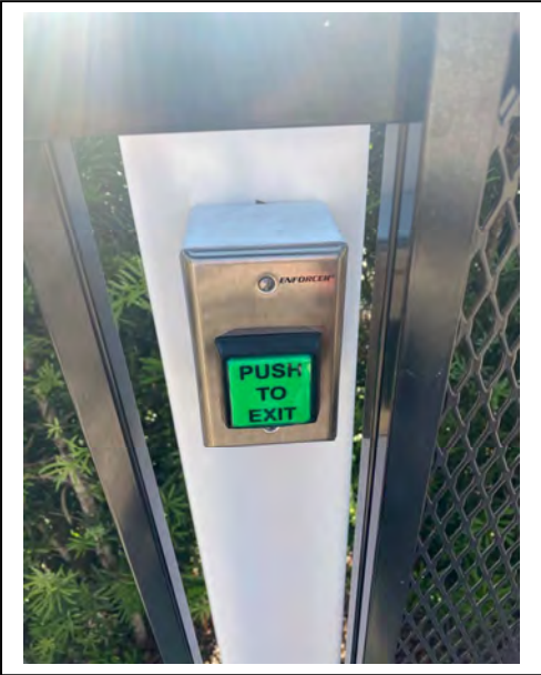
High-Tech Security installed a new Exit release button located at the Pool Deck Parking Entry.
