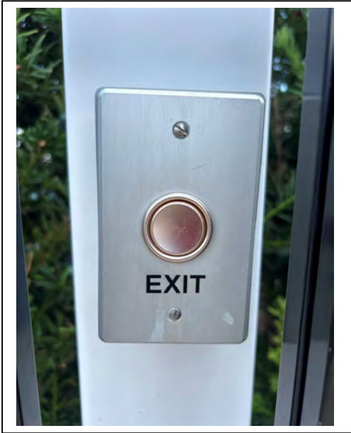
High-Tech Security installed a new Exit release button located at the Pool Deck Parking Entry.
