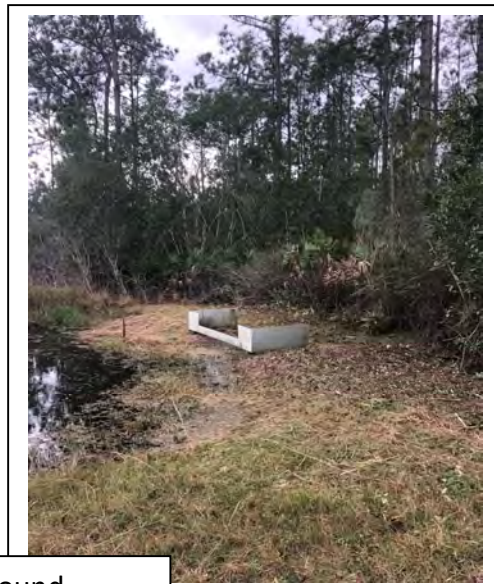
Yellowstone cutback around outfall structure to provide better flow.
